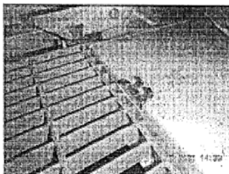
Floor grating hinge broken on second floor entrance.
